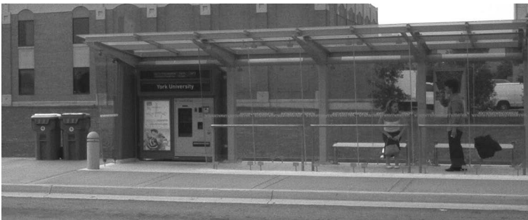
SOURCE: Kittelson & Associates, Inc. EXHIBIT 4-56 BRT Station Example (York, ON)
