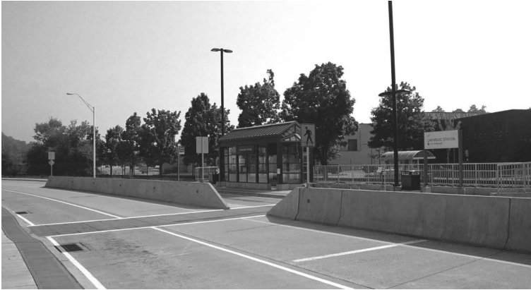
SOURCE: Kittelson & Associates, Inc. EXHIBIT 4-54 BRT Station Example (Pittsburgh)
